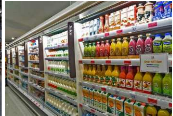
Linear display of milk and fruit juices, displayed on 'Aerofil' equipment. Sainsbury's stores are now equipped with this pioneering technology, which allows a 15% reduction in energy from its refrigerators: a sophisticated technical device in fact prevents cold air from leaving the counter, directing it back into the refrigerator.
