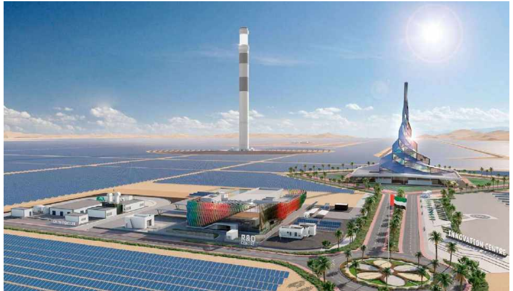
Mohammed bin Rashid Al Maktoum Solar Park. The 900MW sixth phase, which will use photovoltaic solar panels, will become operational in stages between 2025 and 2027. www.khaleejtimes.com
