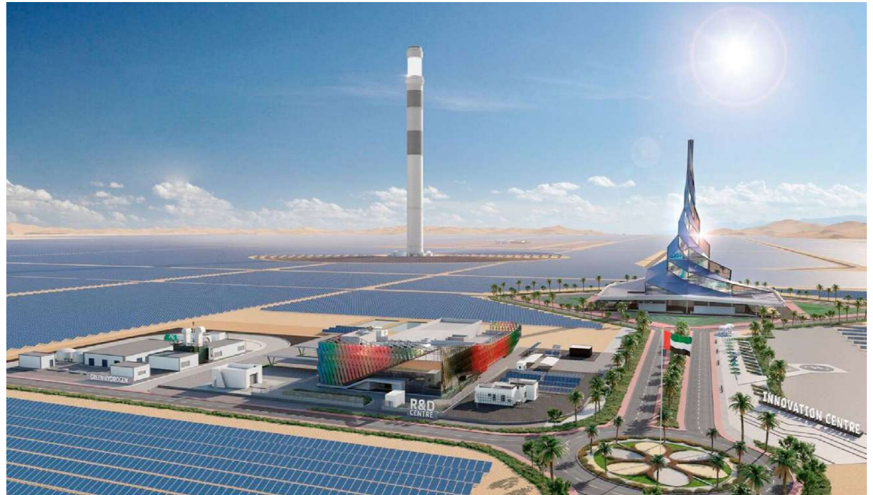
Mohammed bin Rashid Al Maktoum Solar Park. The 900MW sixth phase, which will use photovoltaic solar panels, will become operational in stages between 2025 and 2027. www.khaleejtimes.com
