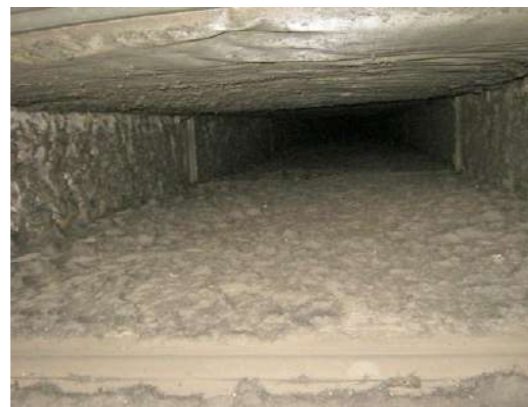
Internally insulated ductwork before & after cleaning.
