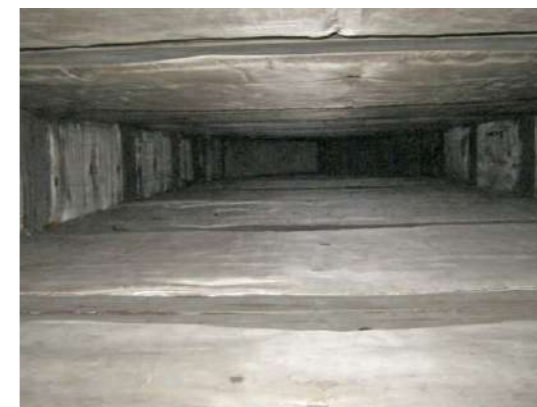
Internally insulated ductwork before & after cleaning.
