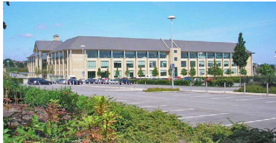
Hilmore House, the headquarters of Morrisons' supermarkets. The name 'Hilmore' is a tribute to Sir Ken Morrison's mother Hilda and was used for a time as a brand name on some of Morrisons' own-label goods. https://en.wikipedia.org/
