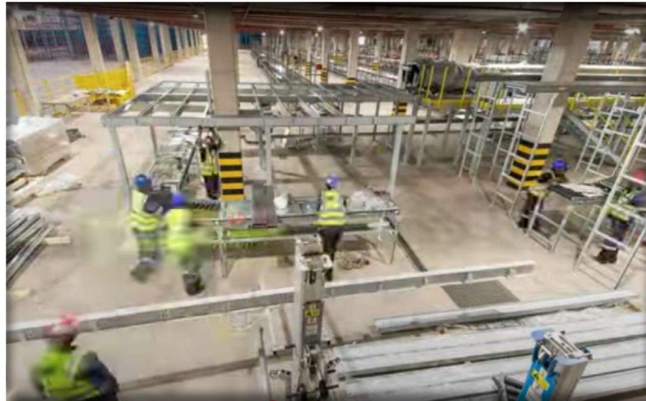
Pepkor KZN warehouse under construction. https://palian.co.za
