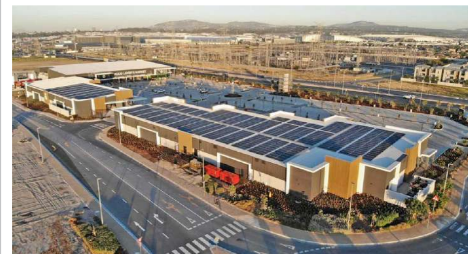
Solar panels ensure that some energy costs for the centre are reduced.
