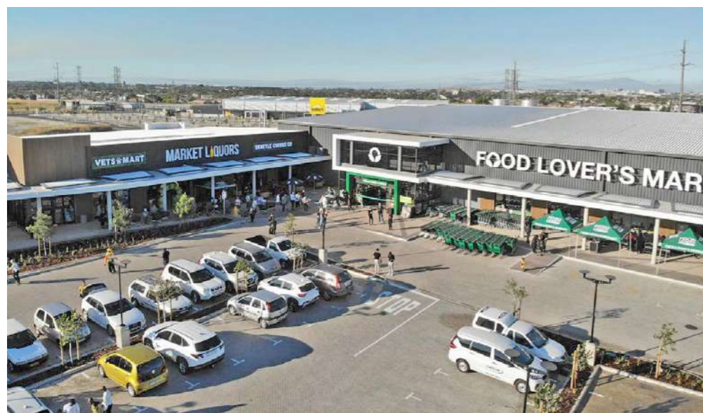
An external view of the store and parking lot.
